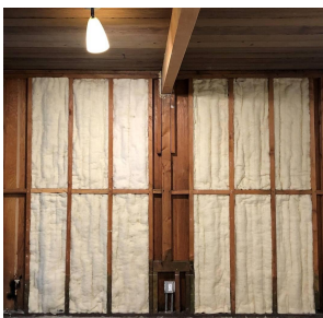
Batts installed in an exterior wall
